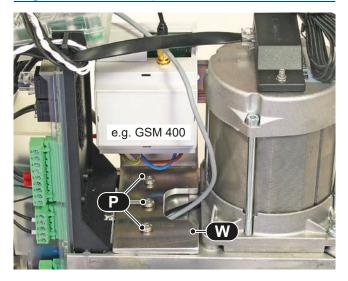
DIN rail without angle: e.g. with ISD and BT40-SO
